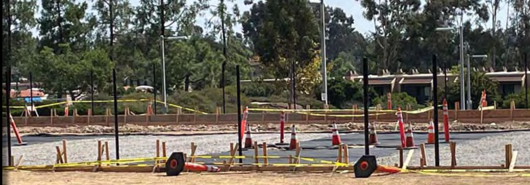
Breaking Ground on Sand Volleyball Courts
